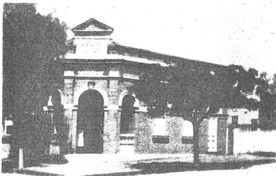
Old Council Chambers, Grenfell. Designed by W.H. Sadlier, Architect whose office is on the left of the Council building. (Supplied by Grenfell Council).
